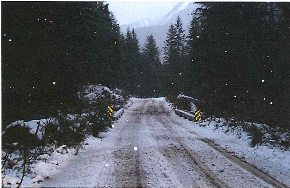
CK-2033 Approach Right Bank
