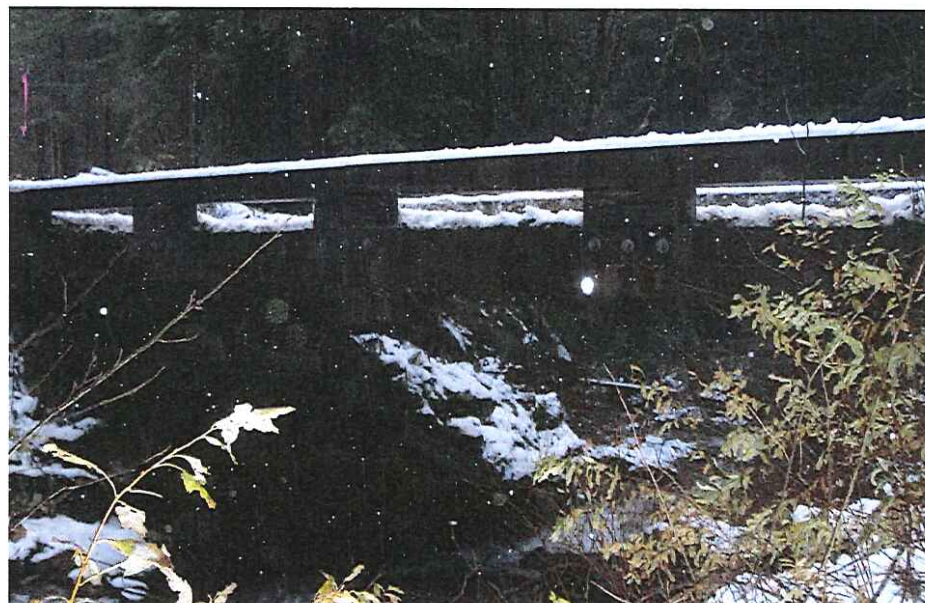
CK-2033 Crossing Upstream
