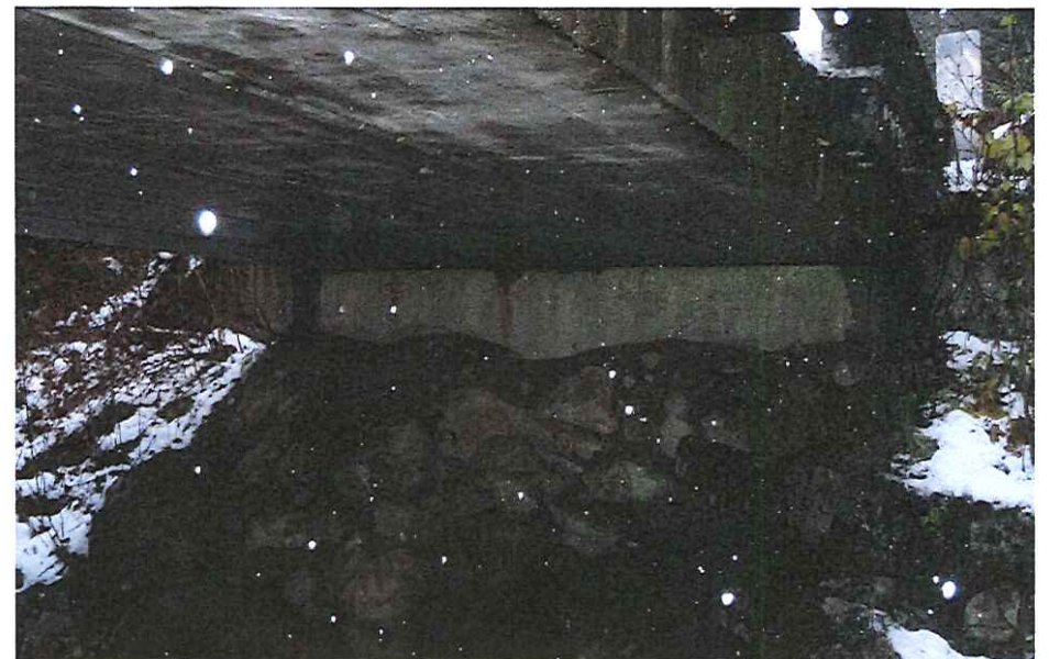
CK-2033 Abutment Right Bank
